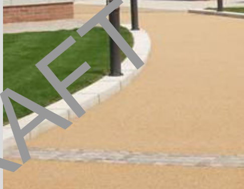
POROUS RESIN BOUND PAVING WITH STEEL EDGE TO ACHIVE CURVES
